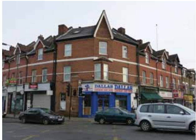
Merton High Street - Merton Road junction
