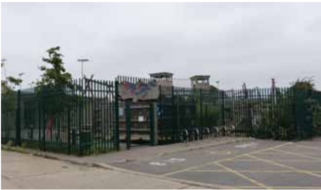
Acacia Intergenerational Centre
