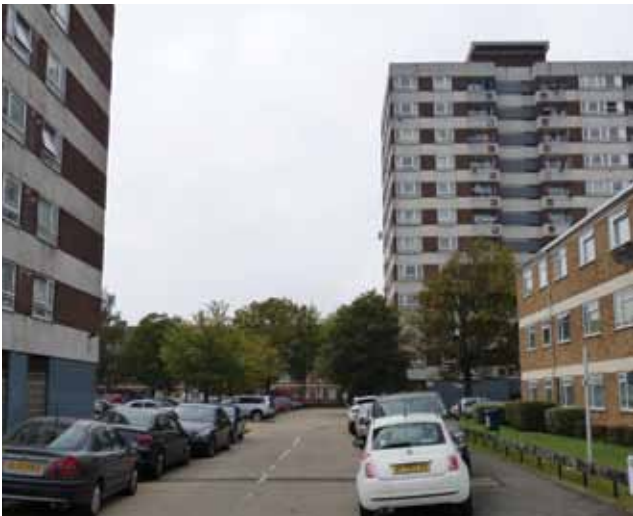
Rear of building block along street frontage
