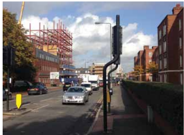
Morden Road (showing Spur House under construction)
