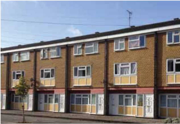
Lack of defensible space
