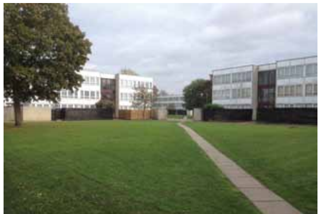
Landscaped interior space
