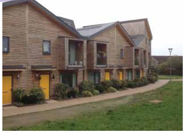
2 storey houses at Rowan Park
