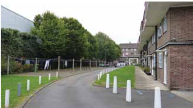
Rear entrances Ravensbury Grove
