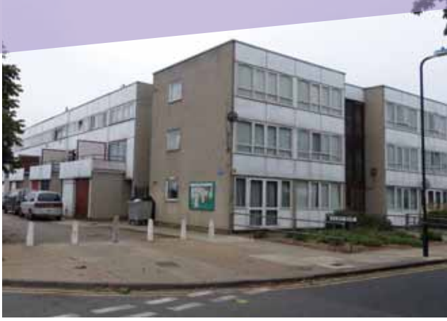
3 storey apartment blocks Eastfields
